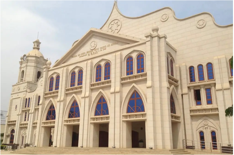
Tocoist Cathedral - Social Administrative Headquarters
